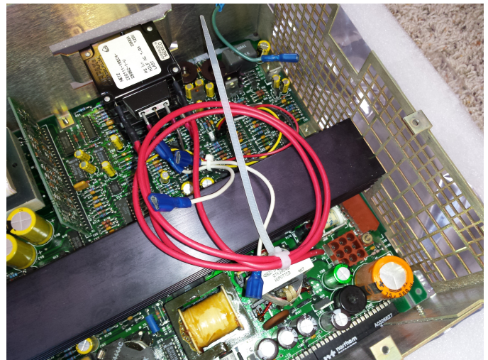
Fig. 18: Secure wires with cable tie
